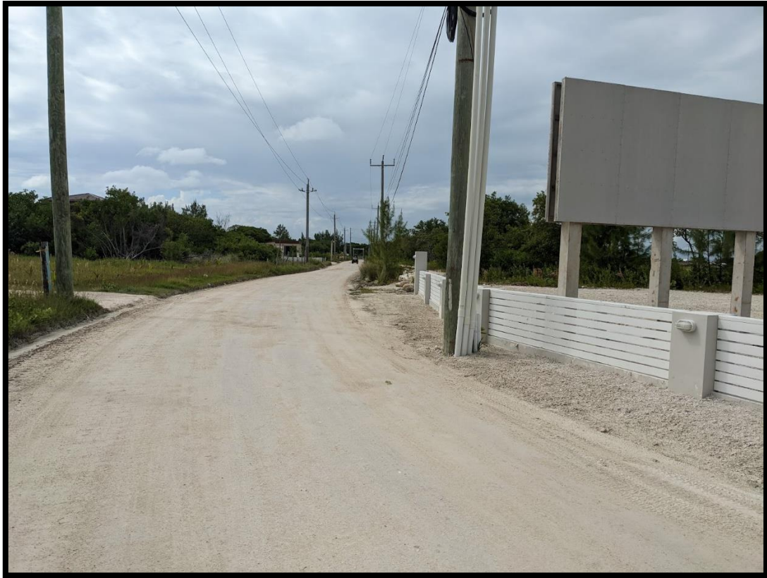
Figure 18 - Initial point of south San Pedro main (Photo: PlanEHS, Nov. 2022)
