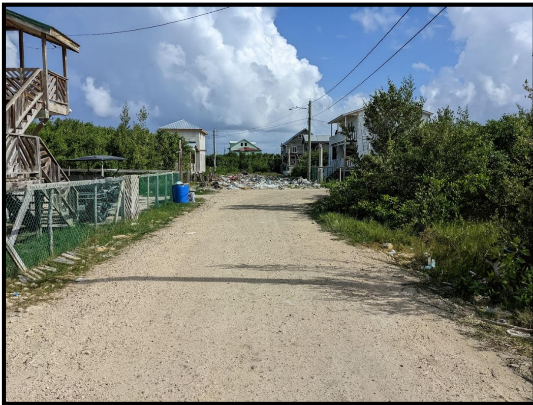
Figure 25 - Micro-dumpsite (front back) on ramification from north San Pedro main (Photo: PlanEHS, Nov. 2022)
