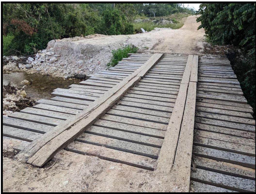
Figure 29 - Drainage canal crossing in easternmost proposed main in Harmonyville (Photo: PlanEHS, Nov. 2022)
