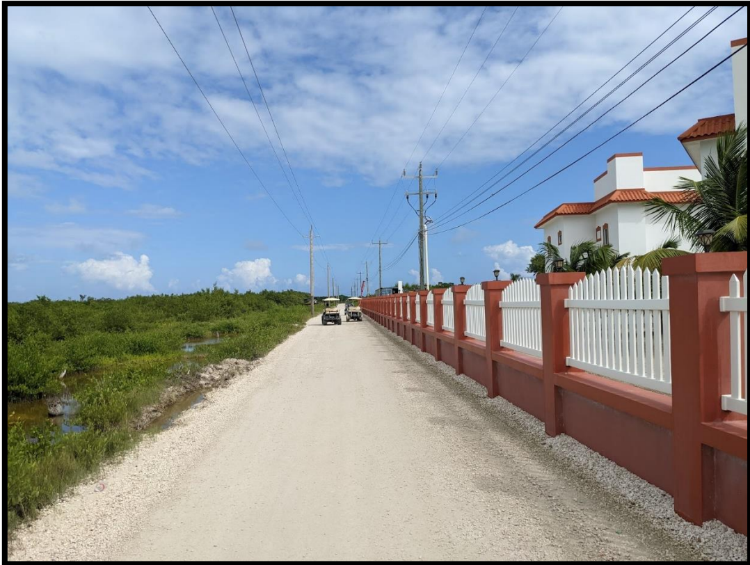
Figure 20 - Lodge / beach resort (Photo: PlanEHS, Nov. 2022)
