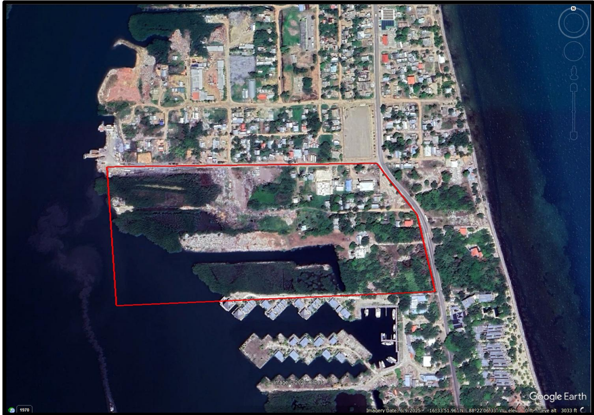
Figure 4 – Potential area for the wastewater treatment plant (WWTP) at Seine Bight. Source: PlanEHS, 2026.
