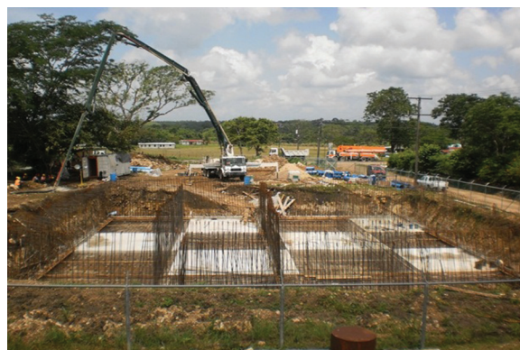
New Belmopan Storage Tank under construction
