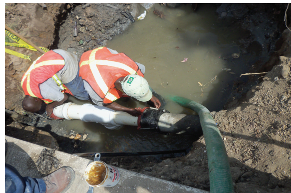
Replacement of aged pipes in progress
