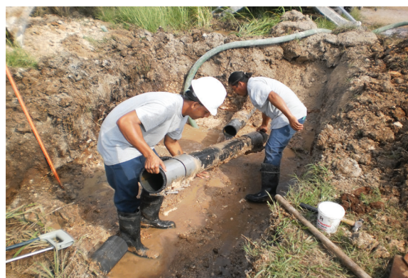
Repair of Water Mains in Corozal
