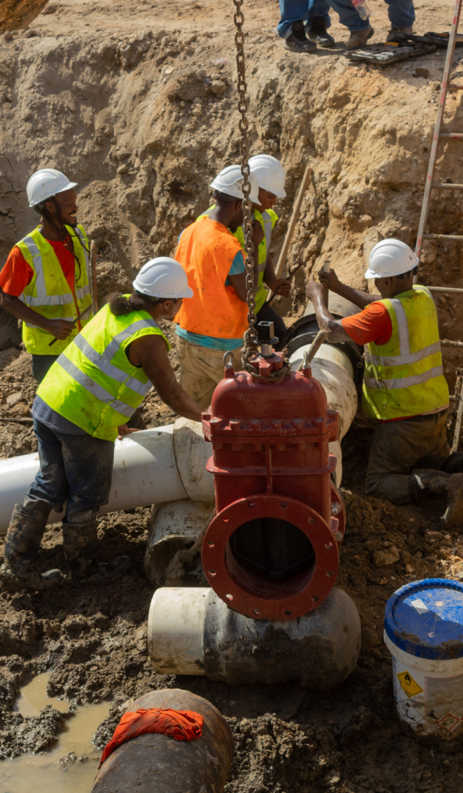
Tie-in of 14" main on Philip Goldson Highway
