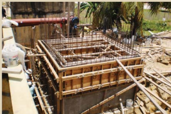
Construction of New Flocculator at Dangriga Water Treatment Plant
